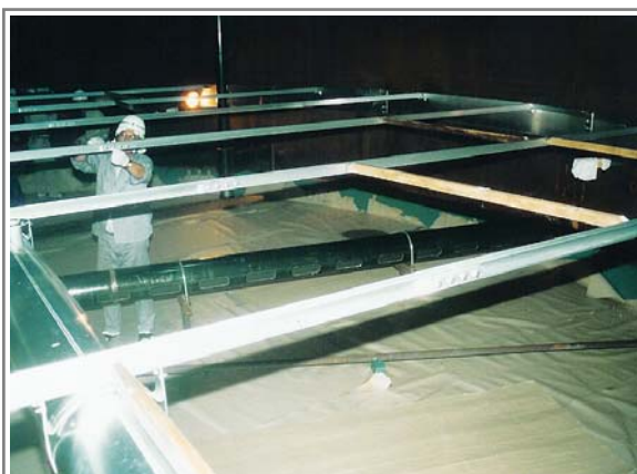
Tubular Pontoon (tube) and Clamp Beam Assembling Works in Japanese Construction Company
