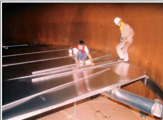
Deck Skin Assembling Work / Japanese Oil Company
