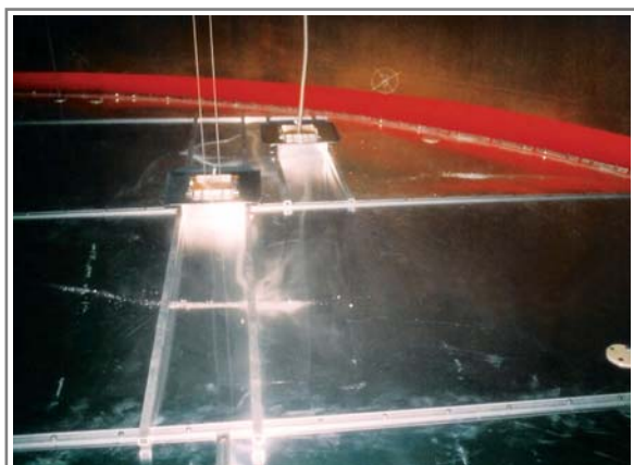
Secondary Wiper Seal & Well Box for Level Indicator
