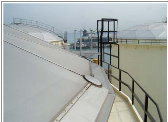
Al. Dome Roof with stair away for the inspection of roof and others P/V vent products
