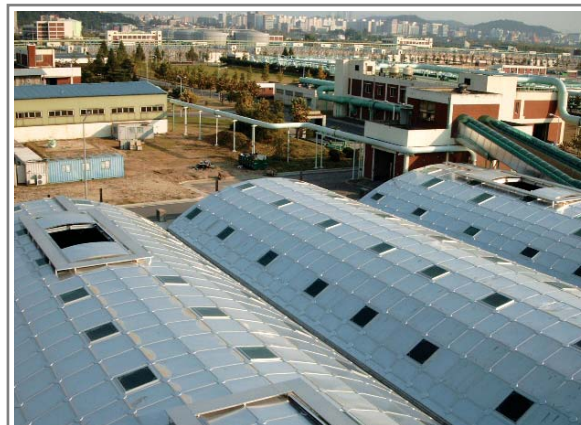
Seonam WWTP AL. Dome Cover (24m, 20m, 20m x 59m) in Seoul City
