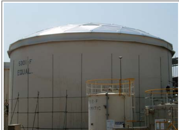
Special Dome flashing & Top angle arrangement works are applied for the above tanks.
