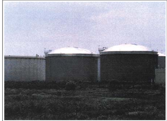
Hyundai oil Refinery's BTX Storage Tank AL. Dome Cover ( \phi 40m, \phi 28m) in Incheon Port City
