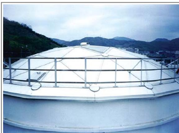
Masan Oil Storage Tank AL. Dome Cover ( \phi 14m) at Masan City in Korea
