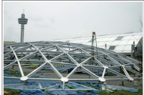
Assembling Main Frame
