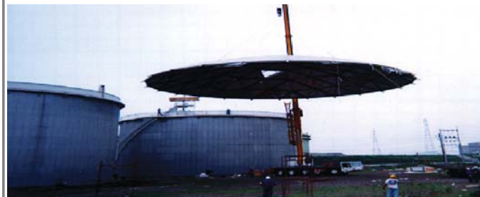
Erection Works of Petroleum Storage Tank Dia. 35m Al. Dome Roof for Local Oil Refinery
