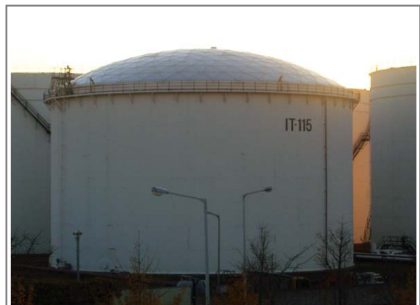
SK Oil Storage Tank AL. Dome Cover ( \phi 34.5m) in Incheon City
