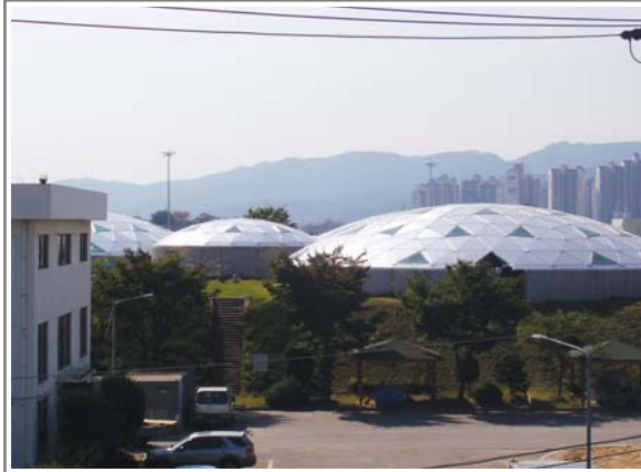
Circular type AL. Dome Cover for Local City Aeration Pond in Korea. Dia 29m and 14m etc
