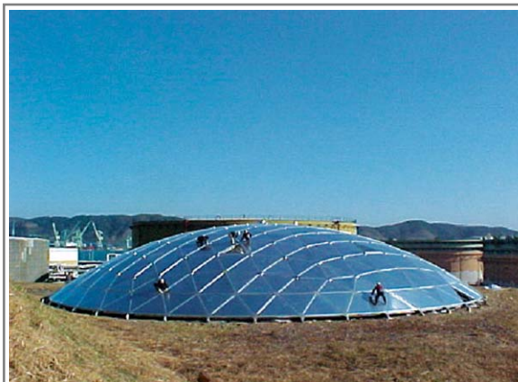
Ground Assembling Works for Oil Storage Tank AL. Dome Cover ( \phi 50m) in Ulsan City. 2002.07
