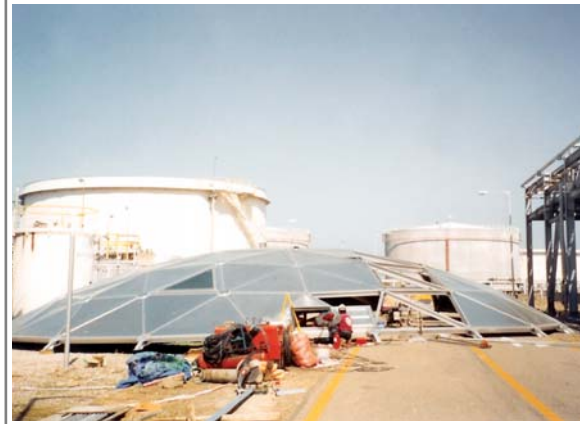
WB, well organized erection crew's final assembling works before Dome lifting works.
