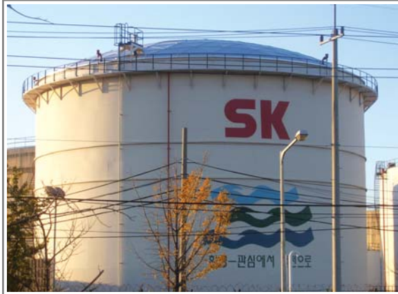
SK Oil Storage Tank AL. Dome Cover ( \phi 25m) in Incheon Port City. 2004.01
