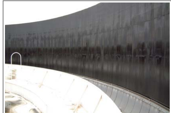
Picture for WB-1 PANTOGRAPH TYPE MECHANICAL SHOE SEAL
