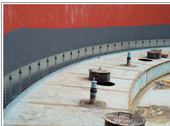
Shoe Plate after Installation
