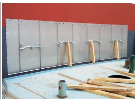
Shoe Plate before Installation
