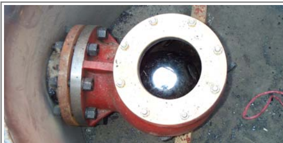
8 inch Float Check v/v is installed in Roof Sump
